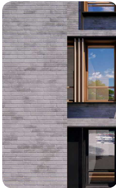
FACEBRICK WORK WITH ALUMINIUM WINDOW BOX FRAMES
